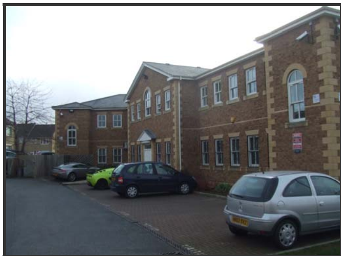
View of Parking Area Outside Main Entrance
